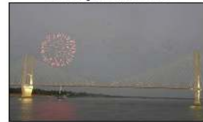
New Greenville Bridge
